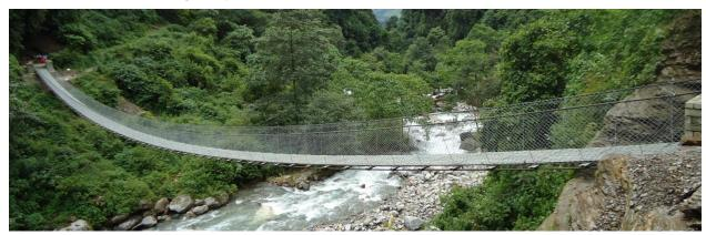
**Suspended bridges** are constructed with steel cables suspended across the river and anchored either side on masonry blocks. They have a walkway that sags in the middle. Such bridges are built in hilly terrain, usually spanning deep valleys, where there is adequate height above the river. A span of this type may go up to 500m.
