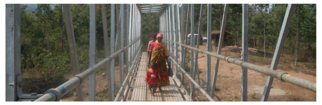
**Pedestrian Steel truss bridges** comprise a rigid superstructure of inter-connected steel elements usually forming triangular units. This type of bridge is only suitable for short crossings and is generally limited to a span of 32 meters.
