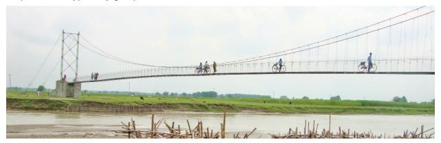
**Suspension bridges** are steel cable structures hung on steel towers either side of the river. They have an upward cambered walkway. This type of bridge is usually built on flat terrain where maintaining enough height above the river would be difficult using a suspended construction. A single span of this type may go up to 350m.
